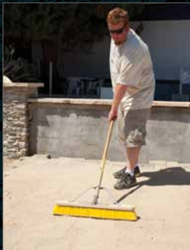
Sweep Finish Sand into Joints
