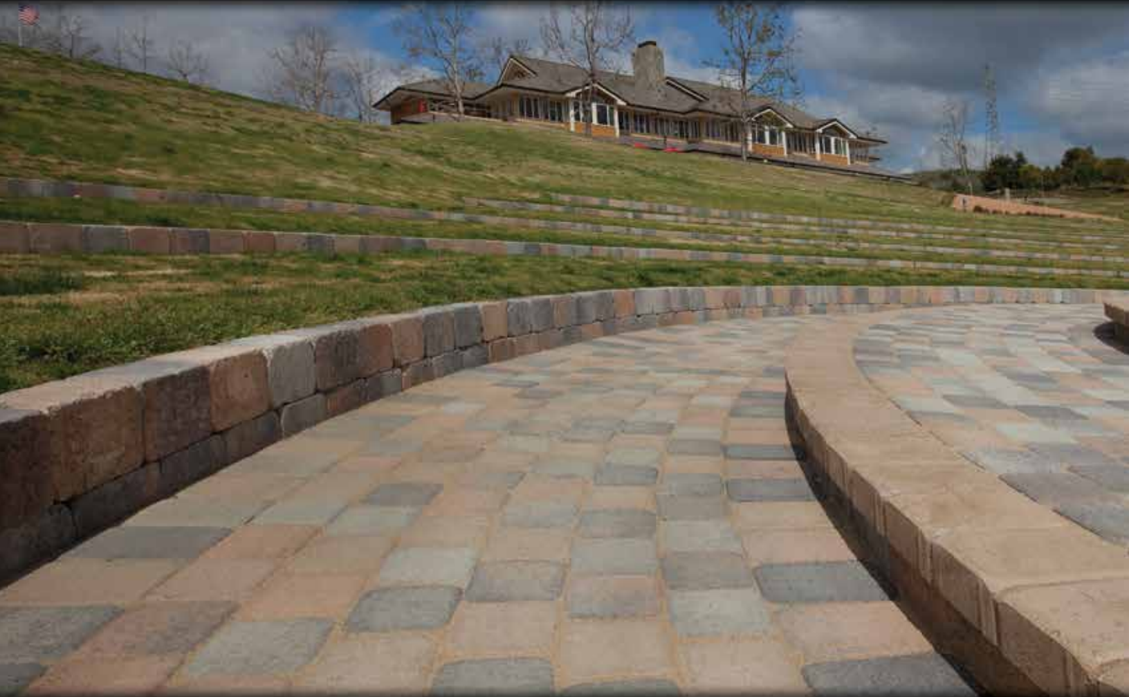
Country Curb Wall tumbled, B6/B7, tight-set mortar (field: Antique Cobble, B6/B7, Random Runner)
